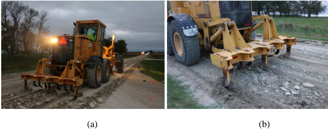
Figure 3.15 Rear ripper resurfaced road surface
