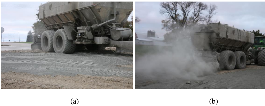
Figure 3.16 Cement spraying (cement)
