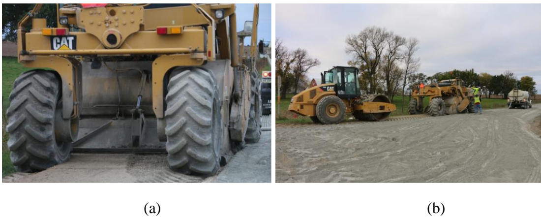
Figure 3.17 Blending with reclaimer (cement)
